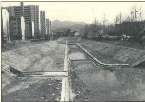
Fig. 1. Riparian zone used as parking lots(left) or blocked by a concrete retaining wall(right).
